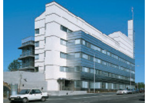
The white ceramic cladding to the central section is attractively contrasted with the stainless steel facade.
