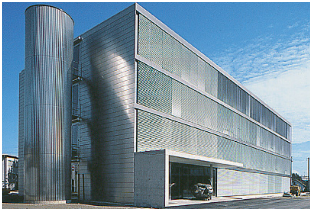
The external sunshading screens the glass facade without affecting the horizontal articulation of the building.
