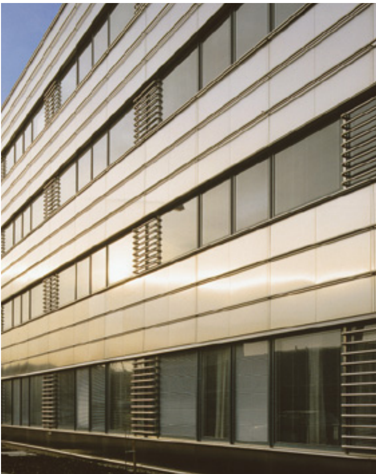
Stainless steel tubes in front of the panels form a projecting plane that articulates the facade.
