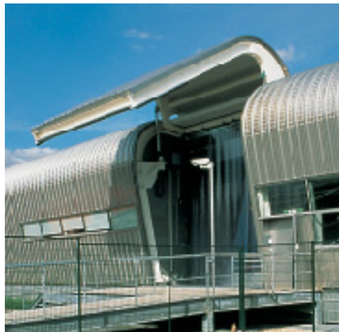
The large entrance door is opened by means of two hydraulically operated screw jacks.
